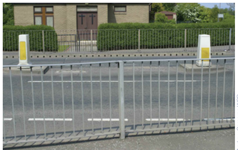
As well as being visually intrusive, the inappropriate use of guard railings can block pedestrian desire lines, with consequential possible dangers
