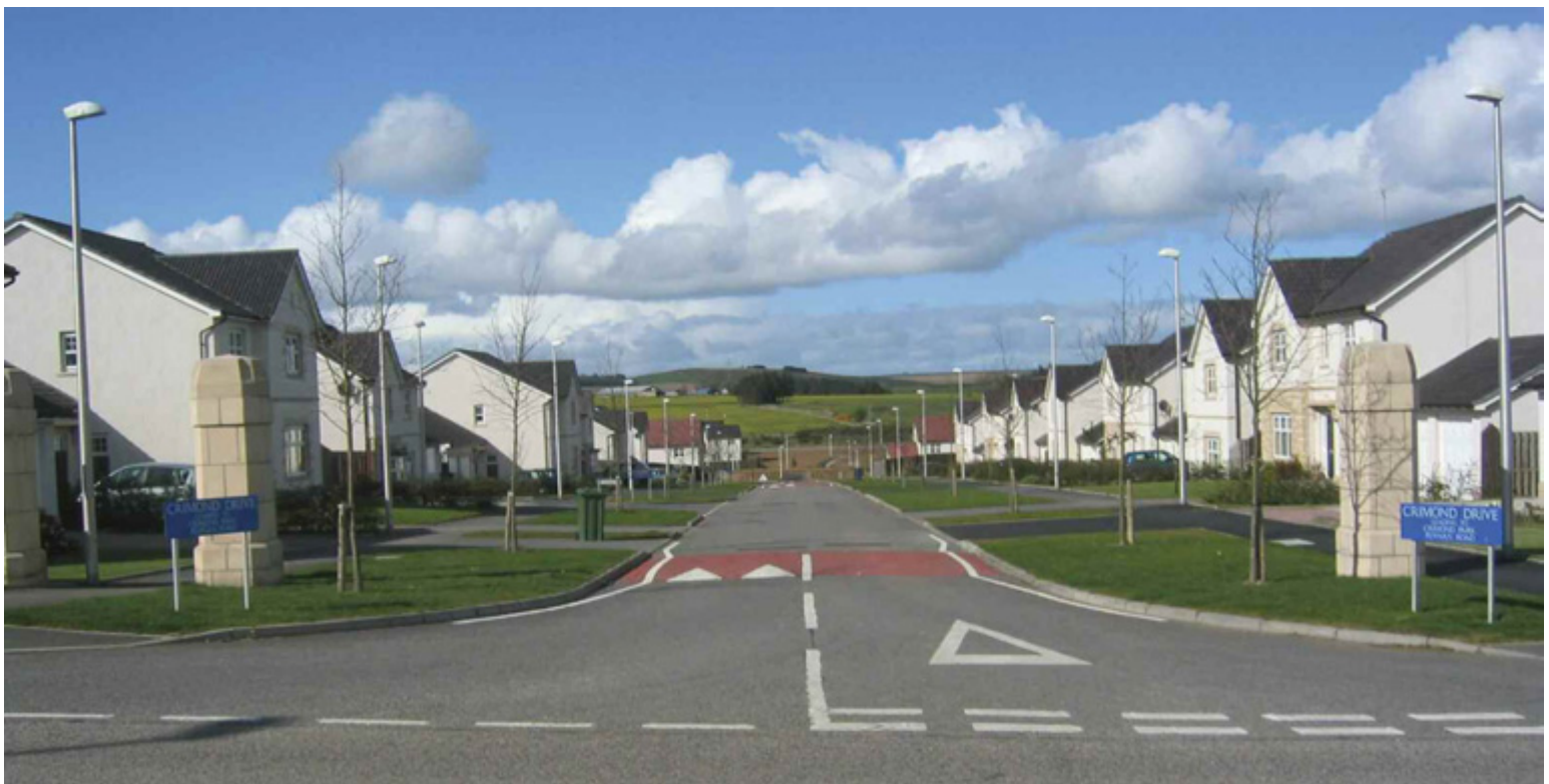
An image of a layout driven by standards and formulaic solutions – the use of large radius bends, overly-dominant lighting columns, large building setbacks, inefficient land use, and inappropriate traffic calming contribute nothing to a positive sense of place
