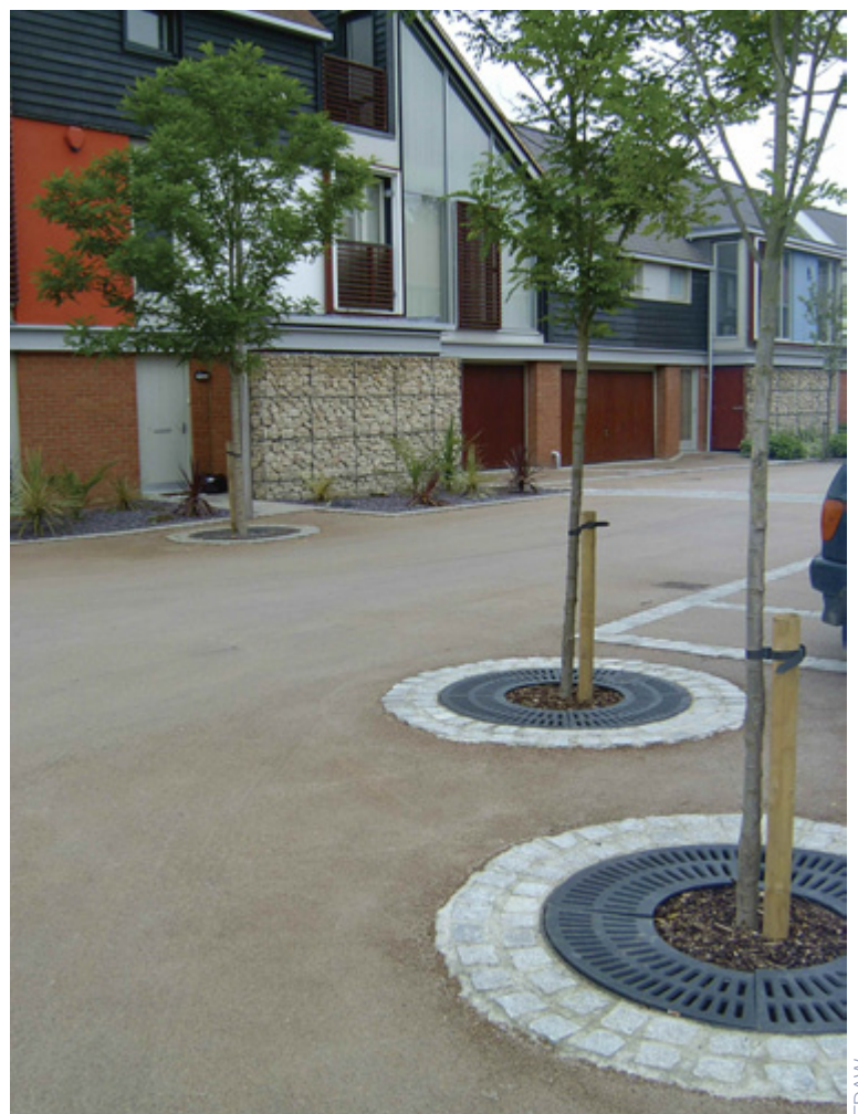
Trees planted in the highway at Newhall, Harlow, help to reduce vehicle speeds
